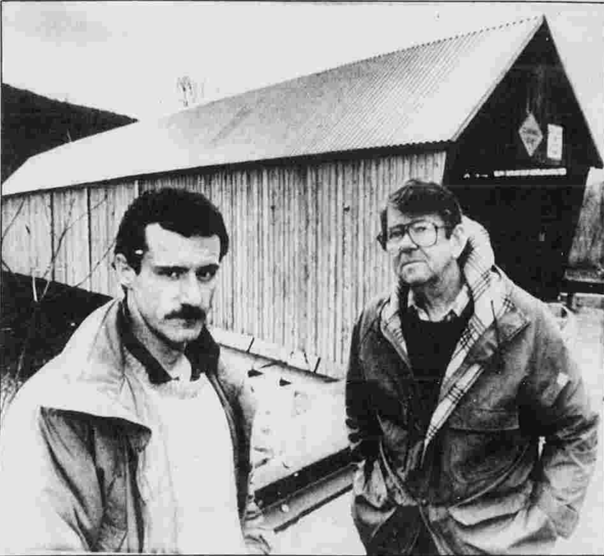
MORE HEAT THAN LIGHT — Dennis DePaull, left, and Harry Francis stand in front of the 113-year-old Lincoln Bridge in Woodstock, Vt. Town residents are upset by the corrugated metal roof with its skylights that was installed in a recent renovation. They want it replaced with a cedar shingle roof.
